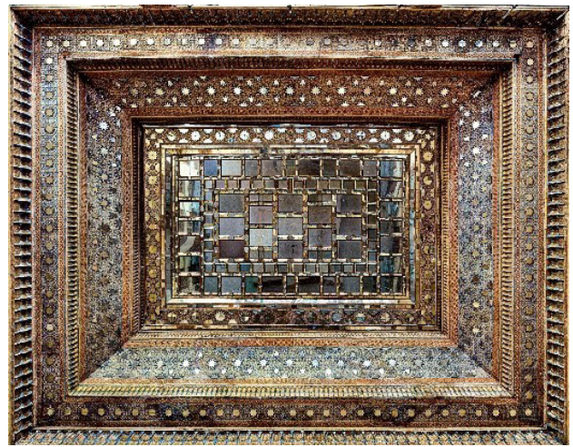
Fig. 1. Installation of big planar mirror (aina Jam) on Chehel Sotoun iwan ceiling, Isfahan, Safavid. Photo: Alireza Sheikhi, 2022.
