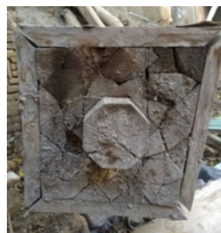
Fig. 10. Layout of Capital Column Shafts. Source: Sina Askari Hassanlouei, 2020.
