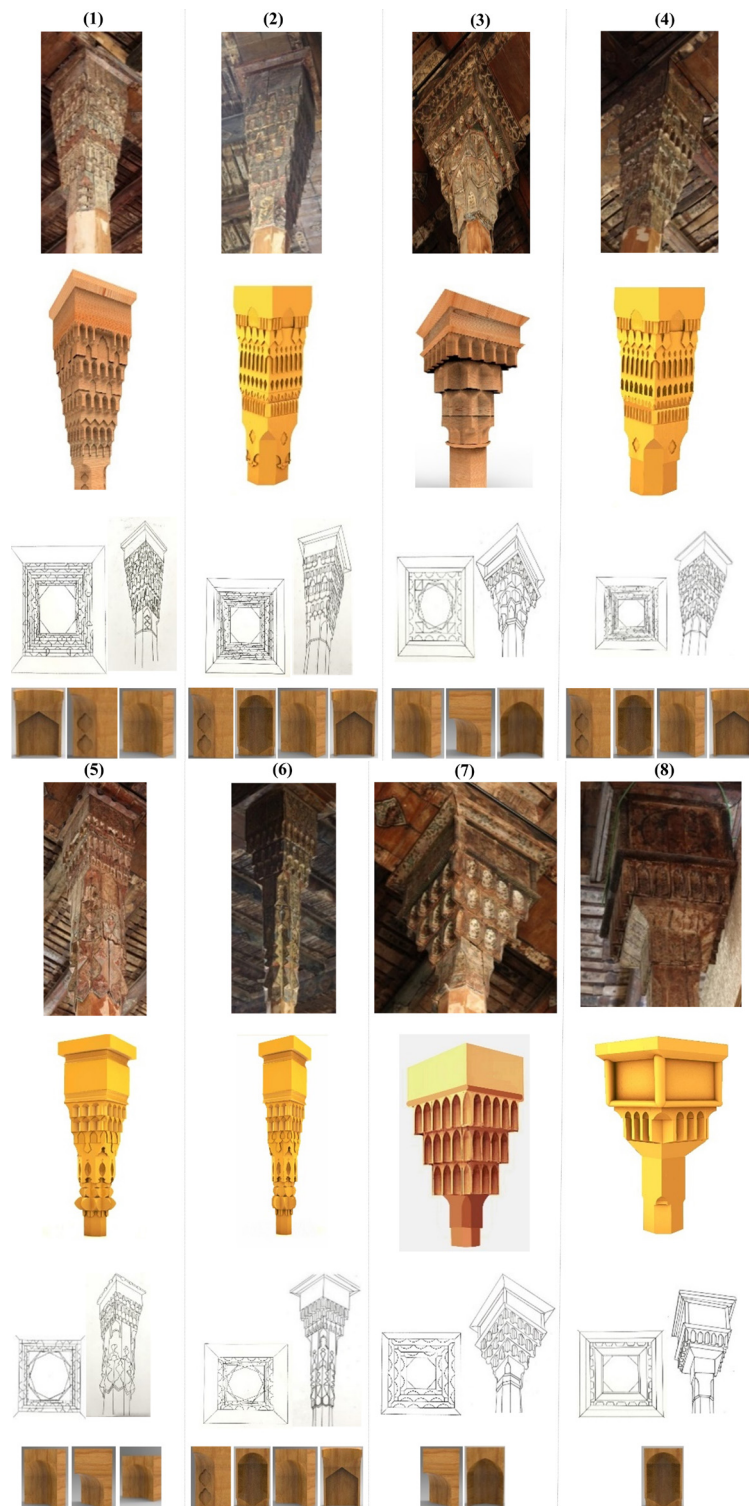
Fig. 2. Introduction of columns of Mehrabad Masque in Bonab; Pieces shaped as symmetrical pillars have been cut and instruments have been placed on top of each other. Source: Authors.
