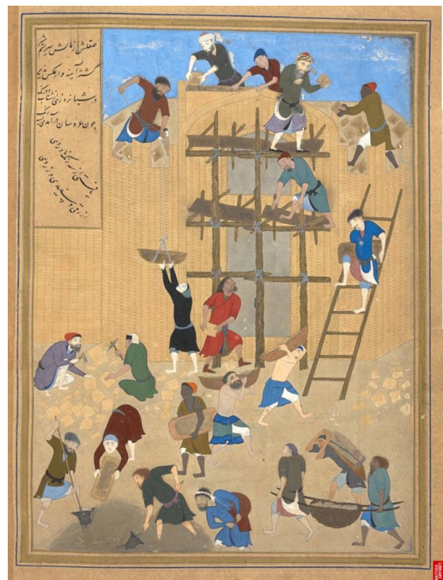
Fig. 1. The depiction of the construction of the Khawarnaq Palace, an artwork by Kamal al-Din Behzad (15th century) in the British Royal Library (or.6810). Source: Gray, 1990, 205.
