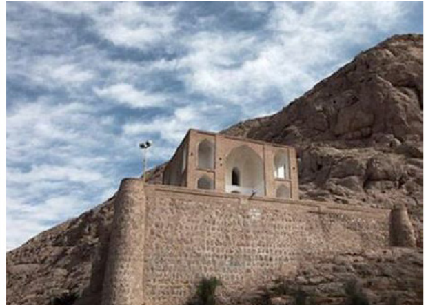
Fig.4. The body of Dargah-Gholi-Beyg that is located at the southern corner of Ghaleh Dokhtar Mountain. Brick is the main material used in construction of this chahartaqi. Furthermore the chahartaqi was built on a number of graves. Source: www.mehrnews.com .
