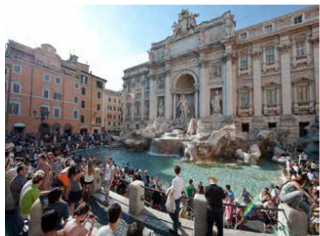
Fig. 5. The development of Trevi's square owing to its biggest fountain in Rome, replacing an ancient aqueduct. Source: https://static.independent.co.uk .
