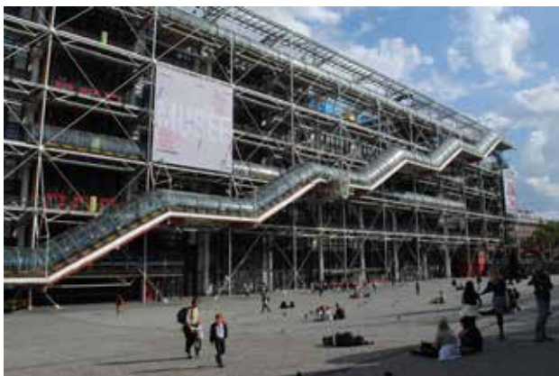
Fig.12. The opposing field of Centre Georges Pompidou; an urban yard active throughout the day and night. Source: Archive of Nazar Research Center, 2015.
