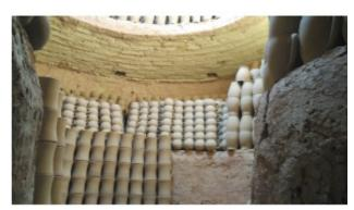
Fig. 2. Outlets used under the niche in the Laljin ceramic kiln. Source: Authors.
