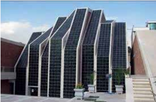
Fig. 4. A mosque in Tehran, Enghelab Street, and the effects of the global model on religious architecture in Iran. Source: http://shabestan.ir/mobile/detail/news/646239 .
