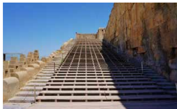
Fig. 19. Temporary floor of Persepolis's stairway prevents the erosion of original stairs. Source: http://www.travelswithdiesel.com/paes/Per2017-
