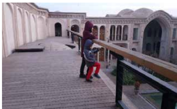
Fig. 18. Temporary floor on the roof of Ameriha inner courtyard. Protective installed parapets ensure child safety. Photo: Elham Andarodi, 2019.
