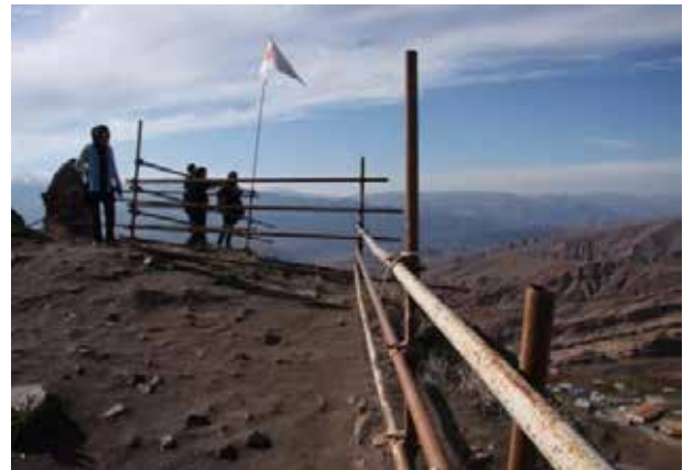
Fig. 14. Scaffolding in Alamut castle. Photo: Betol Sahrakaran, 2009.
