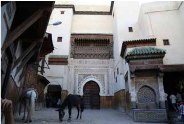
Fig.2.The Najarin Caravanserai and the Sakyah next to it. The main pattern of entrances to the buildings of the city of Fes is clear in this image. This entry is made of lively and decorated samples. Wooded plinth, carvings, and Stalactites, along with Qur’anic verses that are carved on gypsum and wood.
