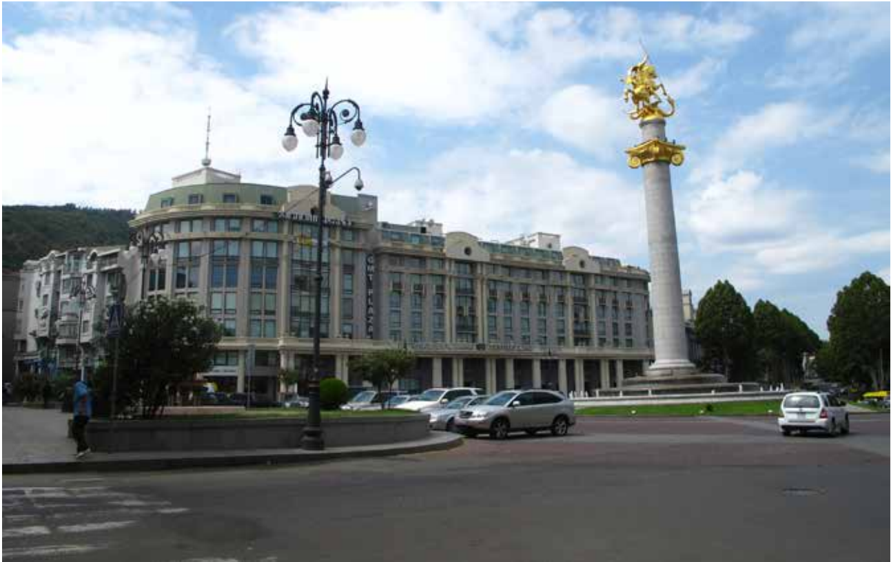
Fig.1. Rehabilitation of historic fabrics with traditional patterns, Freedom Square, Tbilisi, Georgia. Photo: Seyed Amir Mansouri, 2013.
