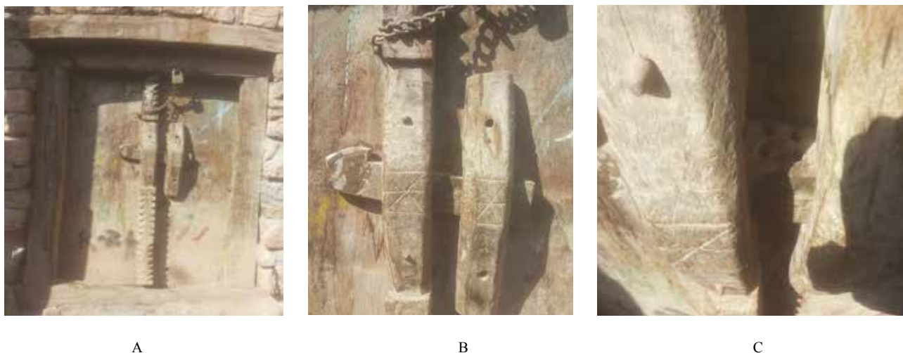
Fig. 4. A: An example of a wooden door in Nowdesheh, B: lock body, C: cipher icon. Source: author's Archive.
